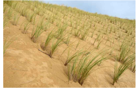
Figure 1: Dunes in Vendée (France) are stabilised by plants of marram grass (image taken from https://www.zoom-nature.fr/loyat-sculpteur-de-dunes ).
